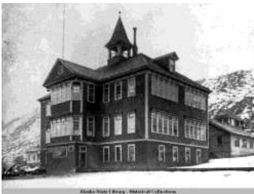
Douglas School, a four-year high school started in 1906; school was destroyed by fire in 1937
